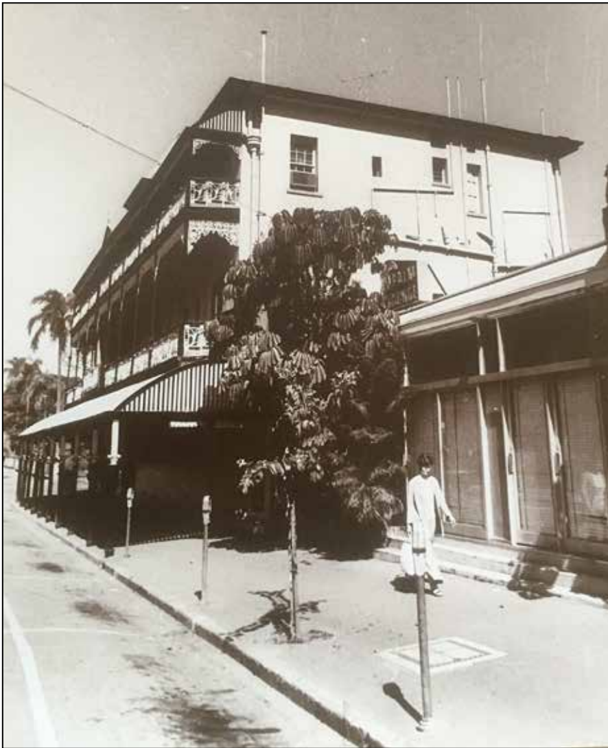
Bellevue Hotel glass-paned area of former beer garden / cottage that Baba used (1960s: photo courtesy Peter Bonenti).
